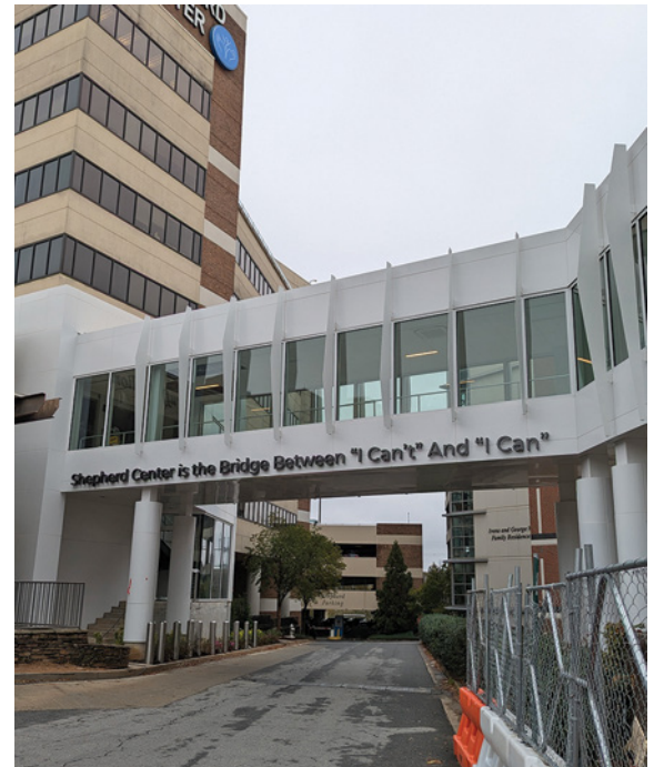
▲ The James H. Shepherd bridge connecting the in-progress Marcus Center for Advanced Rehabilitation to Shepherd Center's existing building
